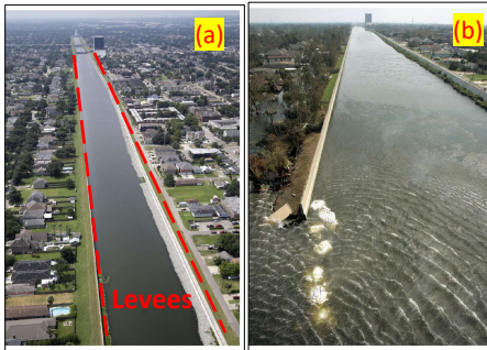
Fig. 1: (a) The levees in New Orleans and (b) the flooding caused by the breach of these levees during Hurricane Katrina.
