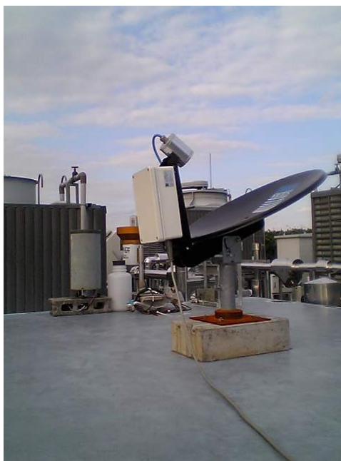
MRR observation equipment on the roof of the Institute of Industrial Science at The University of Tokyo.
