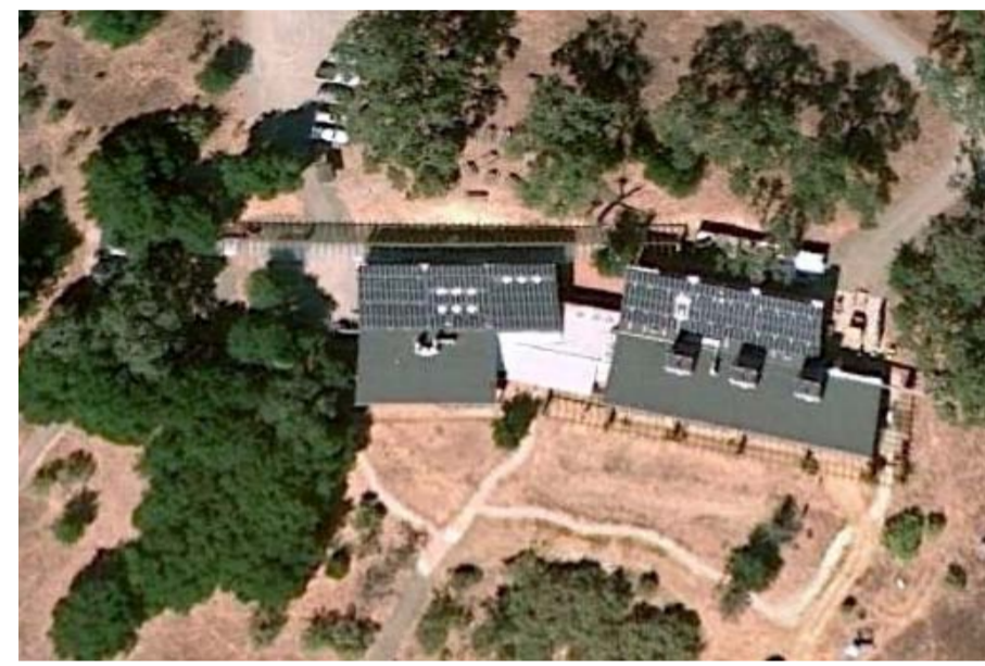
Fig. 3. Jasper Ridge Solar Station
